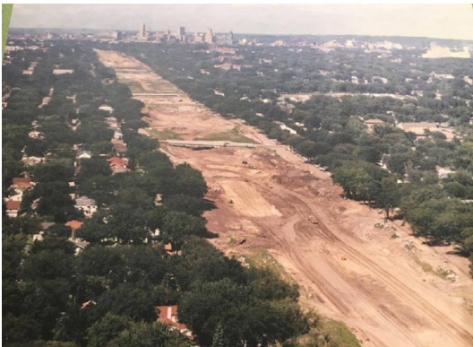
Land Cleared for the Construction of I-35W. Source: Hennepin History Museum.
