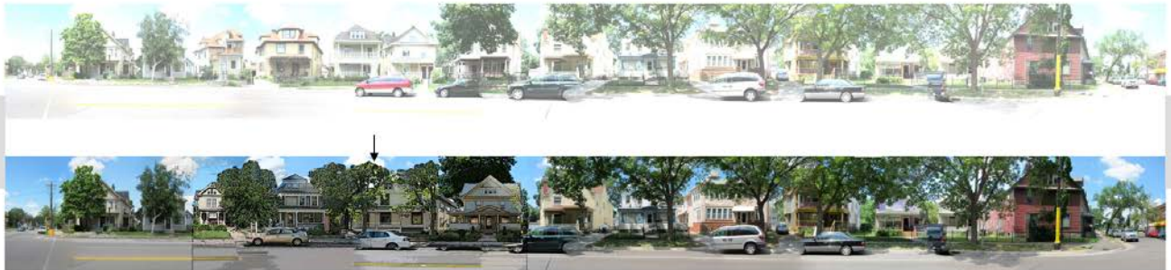
W. 2800 to 2700 BLOCK – Possible residential rehab or conversion to home-office with active street front
