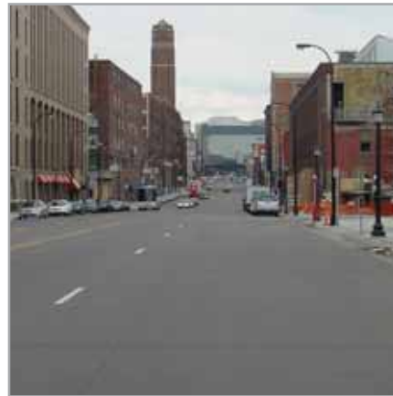
A8 Intersection of Washington Avenue North and Eighth Avenue North.
