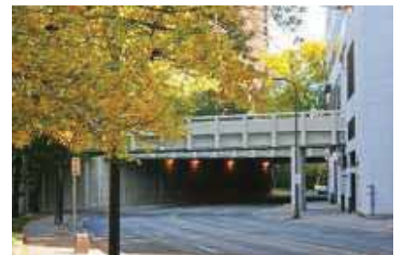
Loring Greenway over LaSalle Avenue
