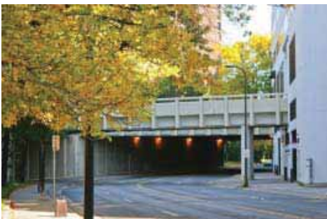
Location of potential stairway connection to Loring Greenway at LaSalle Avenue.
