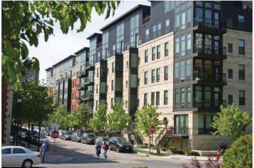
East and north façades of Eitel Building City Apartments, viewed from the entrance path to the Loring Greenway at Spruce & Grand.
