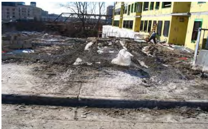
Unmanaged Construction Site with Significant Soil Erosion on Sidewalk and Street
