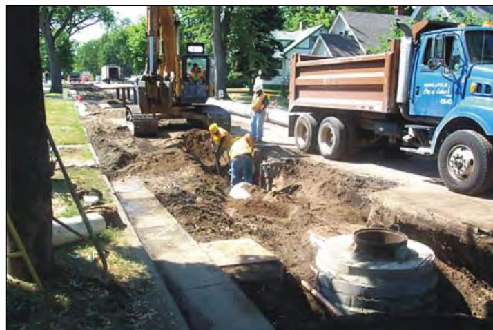
Storm Drain Construction
