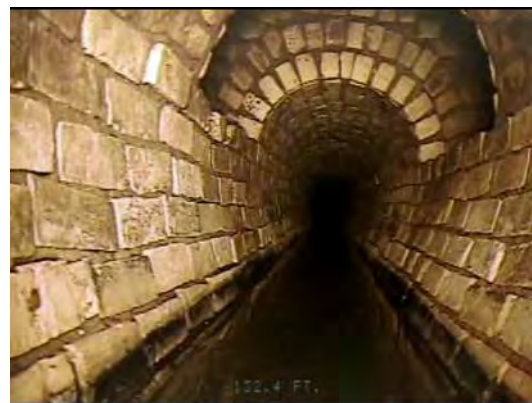
Brick Sanitary Sewer
