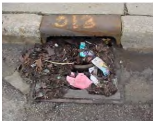
Catch Basin Clogged with Debris
